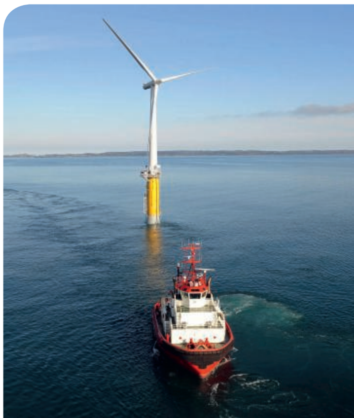
Above: Fixed bottom wind farms are limited to shallow water where steel poles can be driven into the sea bed.
